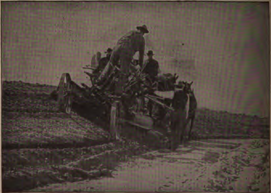
Reclamation Grader Excavating Irrigation Ditch. Figure 13.
